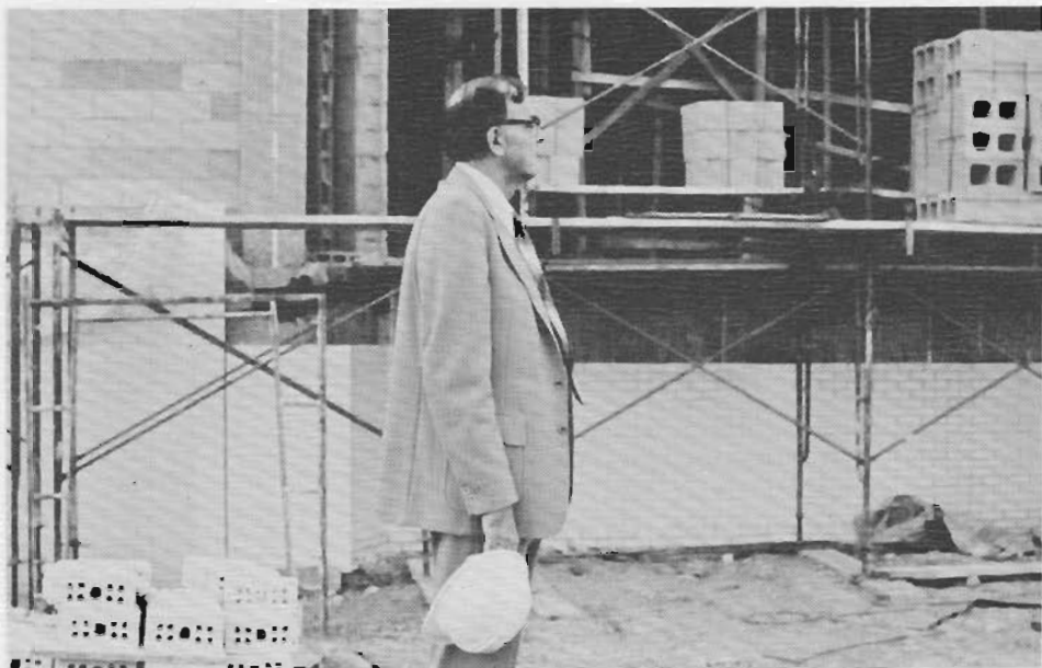
John Green and a dream in progress: Mary Moody Northen Hall.
